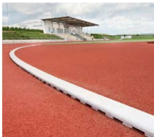
Track Curbing with Drainage
